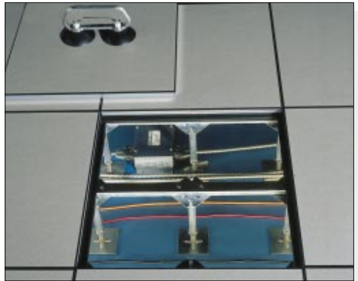
40GGX 12 GR115 HPL06Z2MR15B with additional pedestals on 12" (30.5 cm) centers
